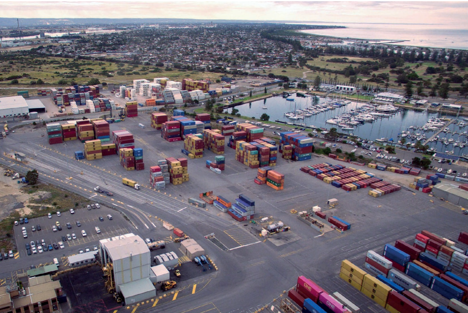
Photo courtesy of Flinders Ports, Australia
